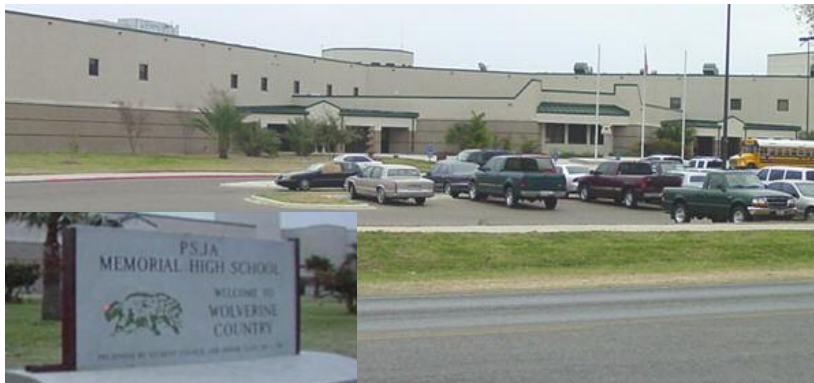
Pharr-San Juan-Alamo Memorial High School's mold problem was resolved with Munters' desiccant dehumidification equipment.
