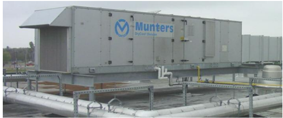
The above Munters system was used to dehumidify PSJA Memorial High School.
